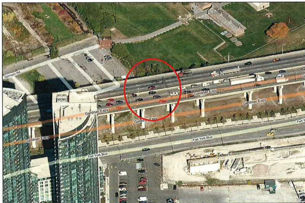
Photo P10 – Aerial Overview of Structure (Bent 85-86) (fair condition – stained and unstained cracking, delaminations and patches)
