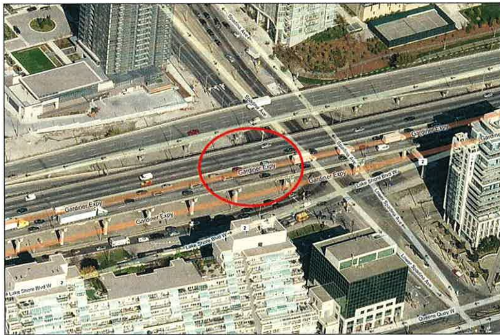
Photo P34 – Aerial Overview of Structure (Bent 131-132) (fair condition – stained and unstained cracking, isolated delaminations and spalls, patches and light scaling)
