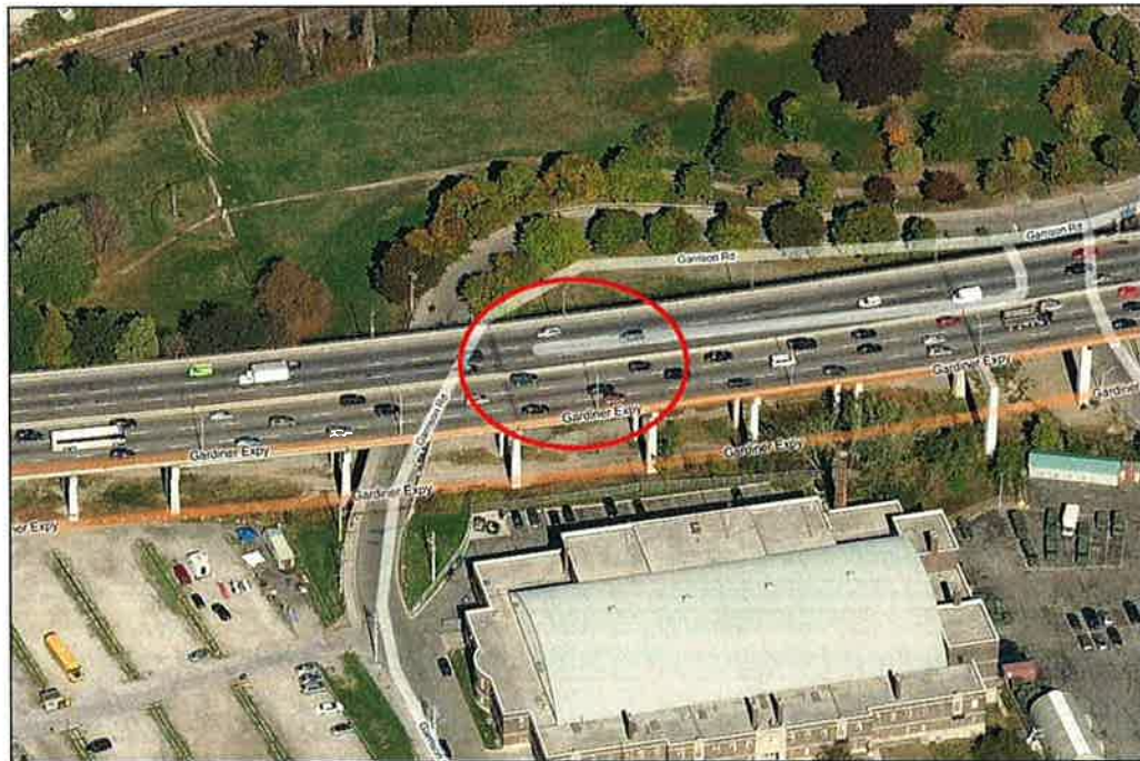
Photo P2 – Aerial Overview of Structure (Bent 53-55) (fair condition – stained and unstained cracking, delaminations, isolated spalls, patches, wet areas and light scaling)
