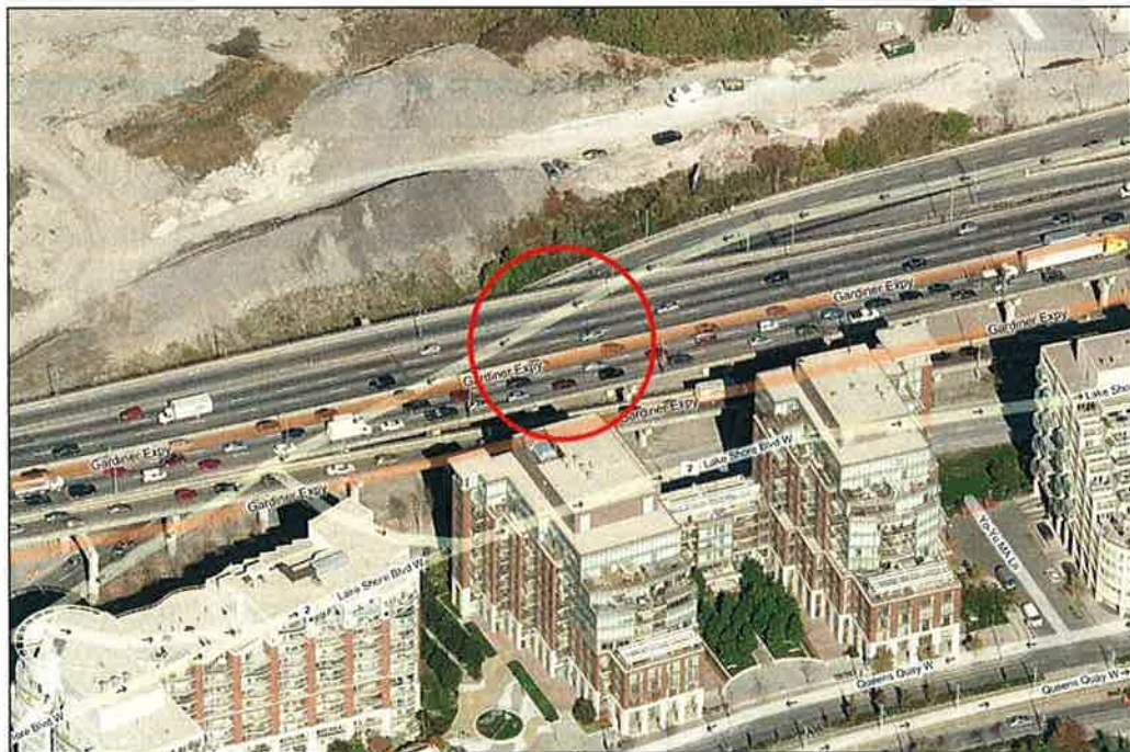
Photo P26 – Aerial Overview of Structure (Bent 120-121) (fair condition – stained and unstained cracking, isolated delaminations and spalls, patches and light scaling)
