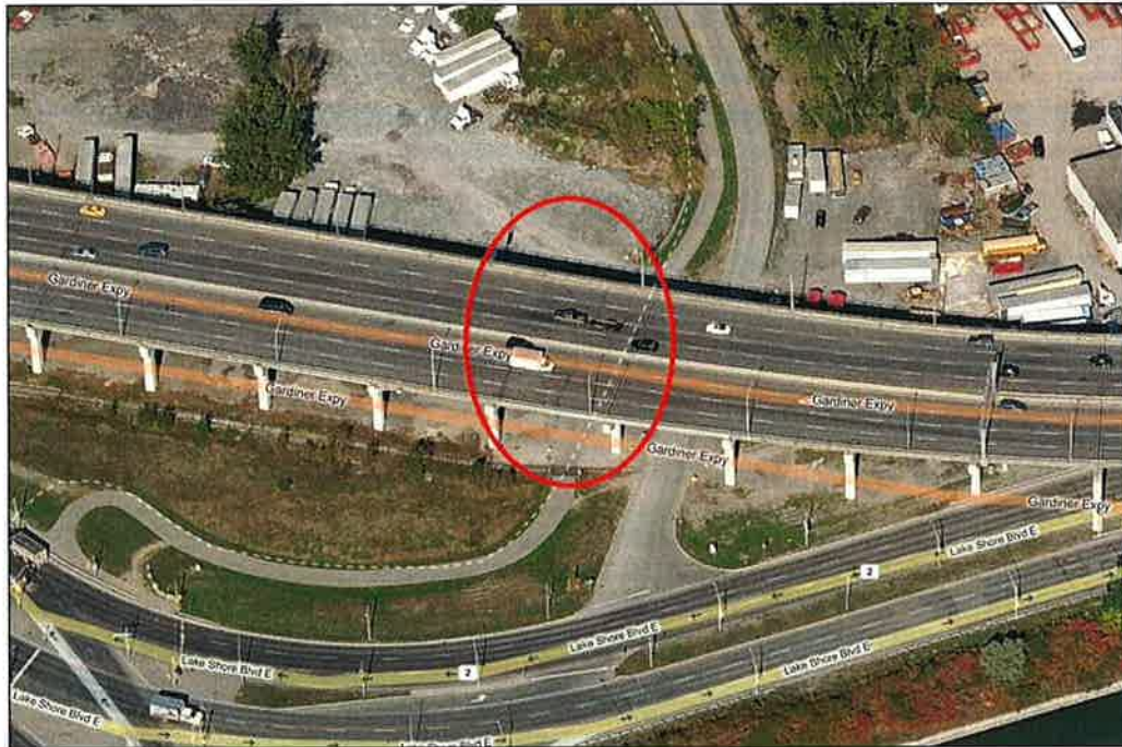
Photo P50 – Aerial Overview of Structure (Bent 306-307) (fair condition – stained and unstained cracking, delaminations, spalls, patches, wet areas and light scaling)
