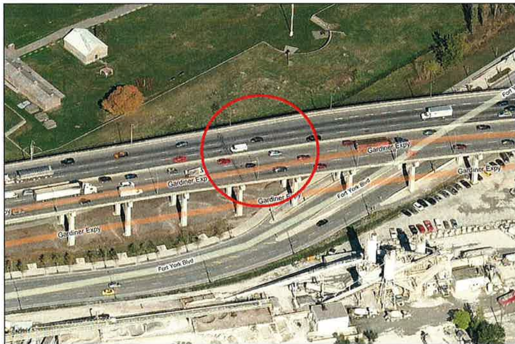
Photo P18 – Aerial Overview of Structure (Bent 91-92) (fair condition – stained and unstained cracking, delaminations, isolated spalls, patches, wet areas and light scaling)
