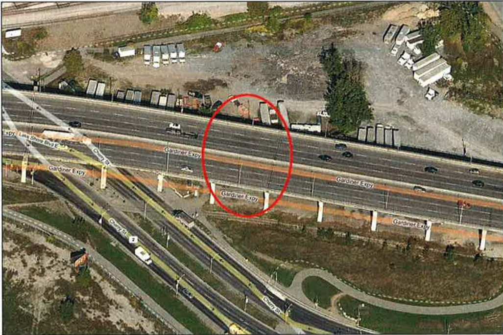
Photo P42 – Aerial Overview of Structure (Bent 301-302) (fair-to-poor condition – stained and unstained cracking, delaminations, spalls, patches, wet areas and light scaling)
